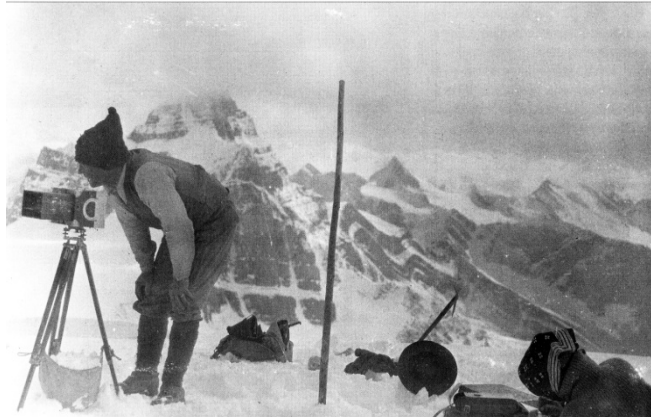
Wheeler's survey crew taking photographs in the Chaba Valley. Notice the bag under the tripod which was filled with snow to weigh the setup down to prevent vibration from wind. 89.03.206, Jasper Yellowhead Museum and Archives.
